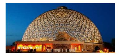
The Desert Dome at the Omaha Zoo is one of the world's largest geodesic domes. It is built from 1344 triangular windows. The base is a regular 96-sided polygon. One can think of this dome as a planar graph with 1344 triangular faces, plus an outside face of degree 96. How many edges and vertices does this graph have? Approximately what is the average degree of the vertices?
